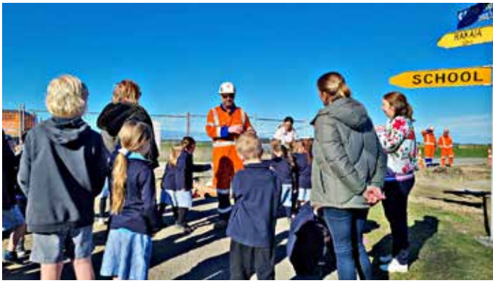
Lauriston School visit the site and speak to Dave Rowlands, Project Manager, ACL about the work being done and the importance of traffic management and road safety.
