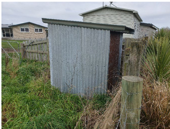
P5: Small "pump" style shed along south-western boundary.
