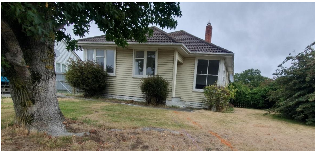
Photograph B10: Front (north-eastern) elevation of dwelling (facing south-west).
