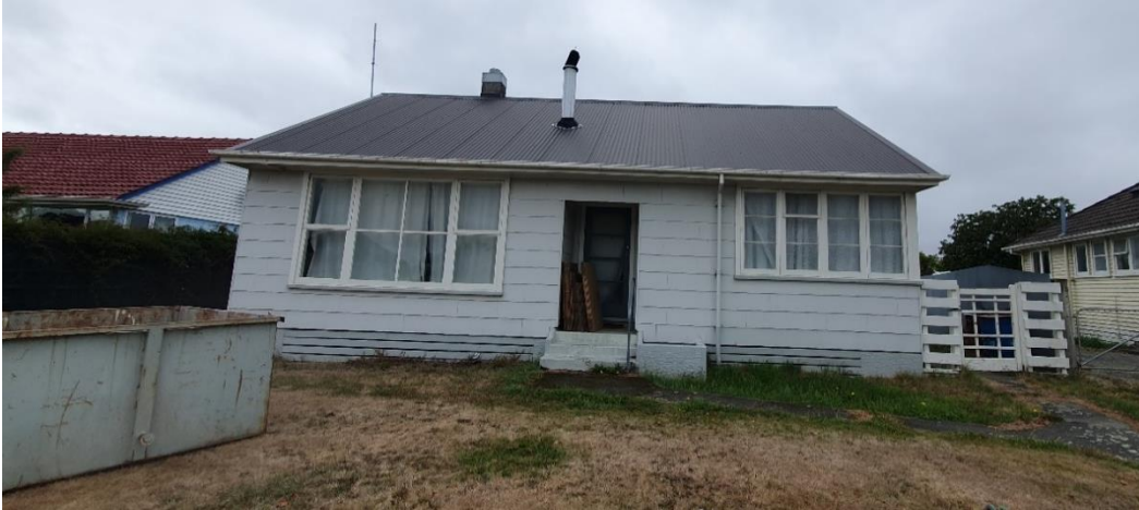
Photograph B1: Front (northern) elevation of dwelling (facing southwest).
