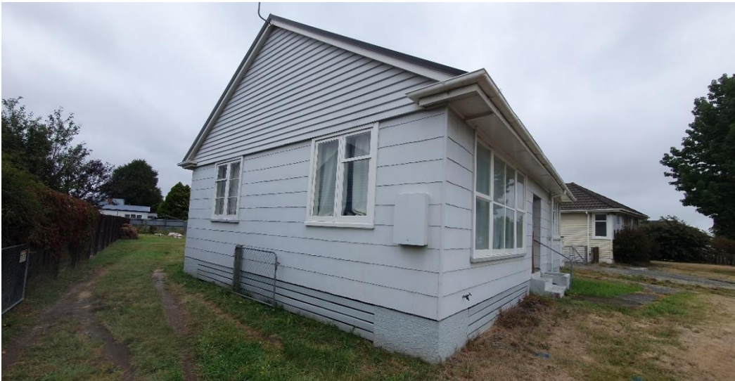
Photograph B2: front and side (south-eastern) elevations of dwelling (facing west).
