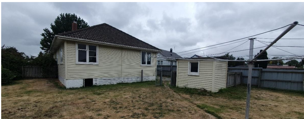
Photograph B14: Shed and southern elevation of dwelling (facing north-east).
