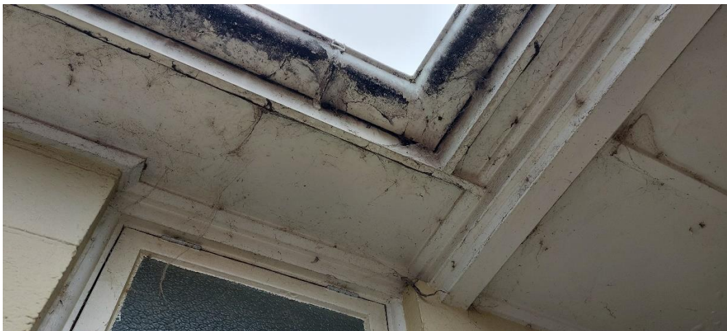
Photograph B22: Soffit detail (PACM cement sheet).
