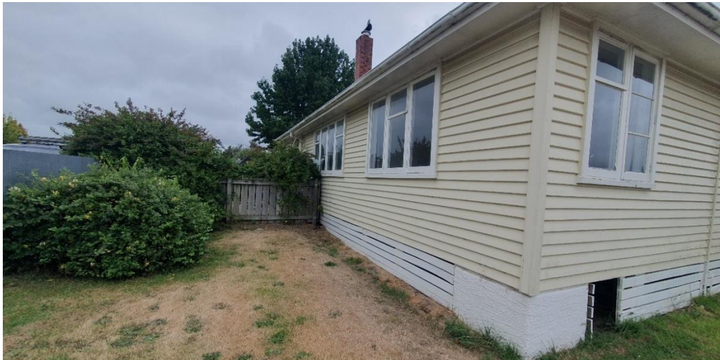
Photograph B12: Rear and north-western elevation of dwelling (facing north-east).
