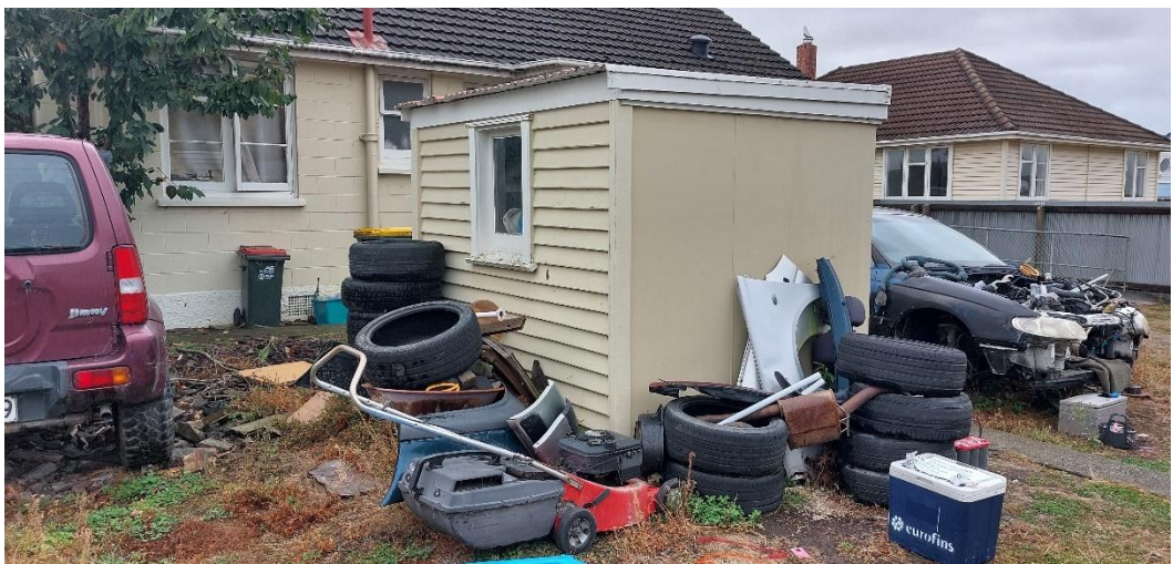
Photograph B21: Shed detail (facing east). Weatherboard and PACM cement sheet cladding. Stockpiled tires and car parts next to shed.
