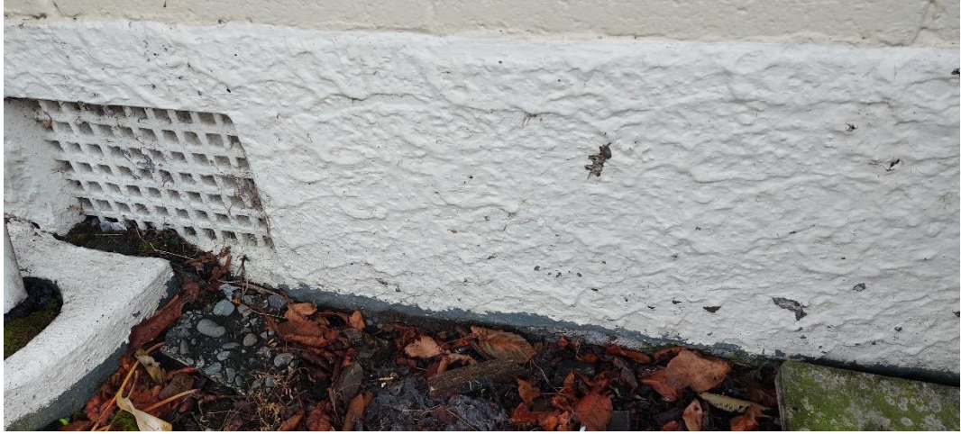
Photograph B23: Dwelling foundation detail (textured PACM (stucco) render).
