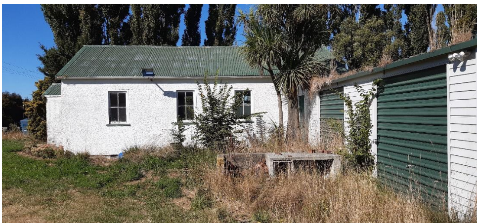
Photograph 3 – North Elevation of Scout Hall and frontage of Sheds
