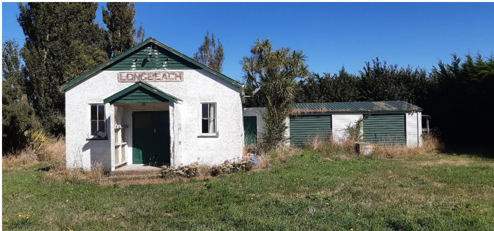
Photograph 1 – East (Roadside Elevation)
