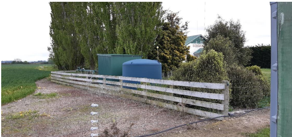
Photograph 5 – Neighbours' Pump Station
