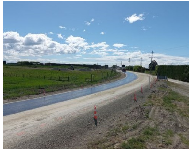
Sealing – Pudding Hill Rd
