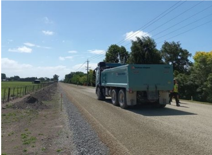
Basecourse construction – Beach Road East
