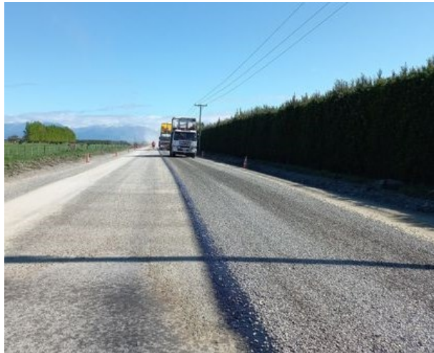
Sealing – Ashburton Staveley Rd
