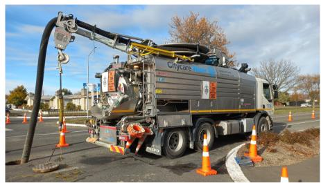
digging up a pipe to inspect it. Some of the pipes being inspected will be glazed earthenware installed in the 1920s.
