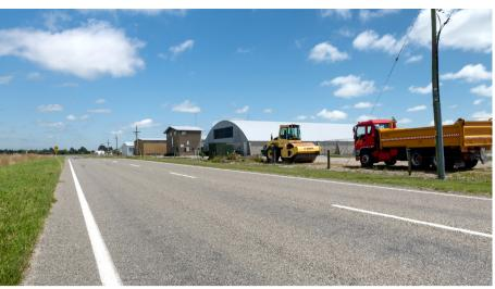
"This is an older sealed road, so the failed areas will be dug out and a new layer of basecourse placed to better cope with the volume and weight of traffic that uses it today."
