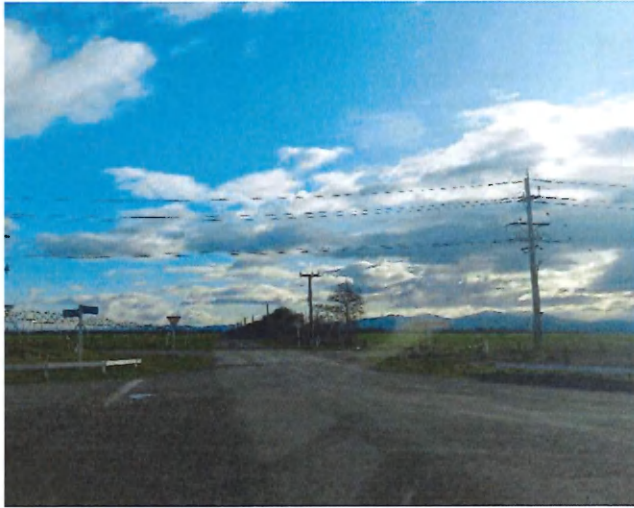
Upgrade to Poplar Road and Coldstream Road –
