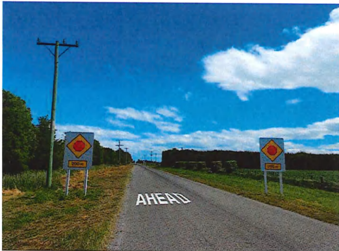
Upgrade to Methven Chertsey Road and Lyndhurst Road –
