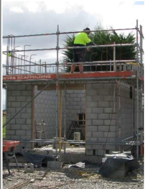
Tinwald WTP UV Upgrade
