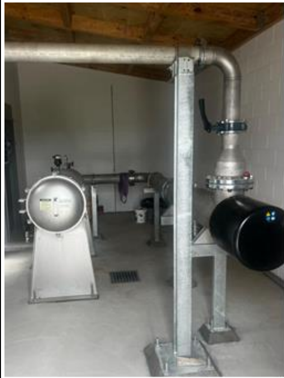
Hinds WTP UV/Filtration Upgrade
