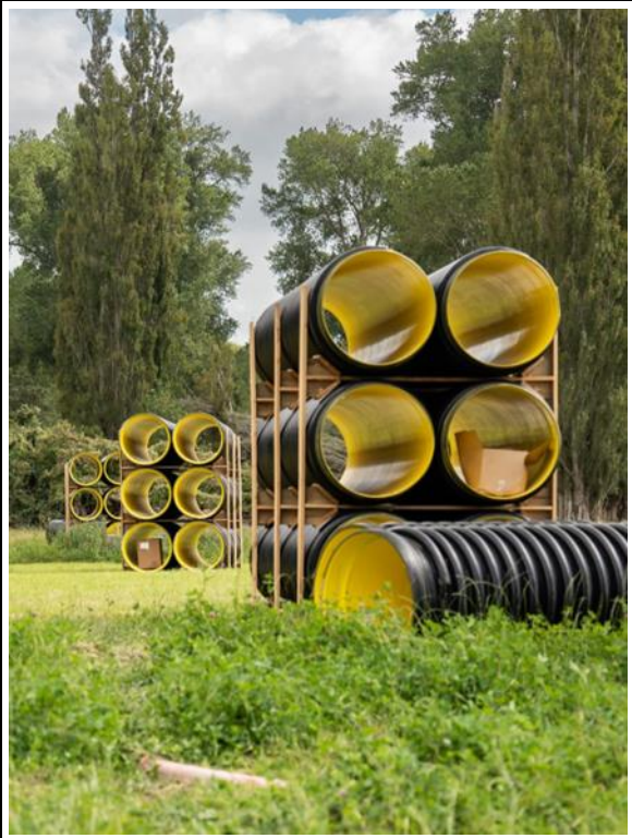
Grit Chamber Pipeline Renewal
