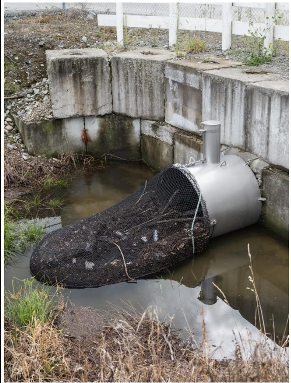
Kermode St Stormwater trash sock
