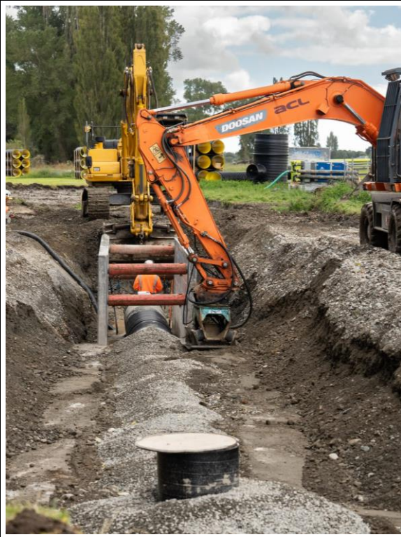
Grit Chamber Pipeline Renewal
