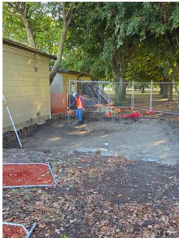
Argyle Park WTP UV Upgrade
