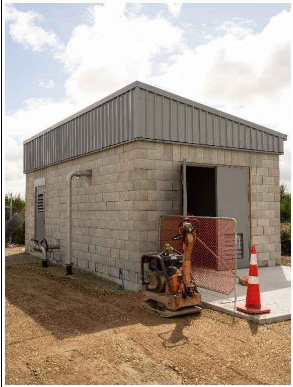
Hinds WTP UV/Filtration Upgrade
