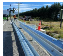
W Section Guardrails 133 each
