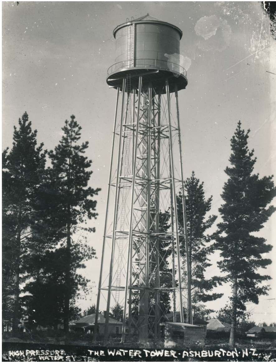
Figure 5 Water tower in Ashburton, image not dated
