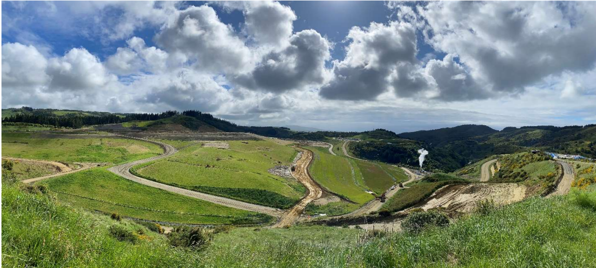
Panorama of the Kate Valley operation with a plume of water vapor above the new landfill gas fueled leachate treatment plant. Tiromoana Bush and the Sea beyond
