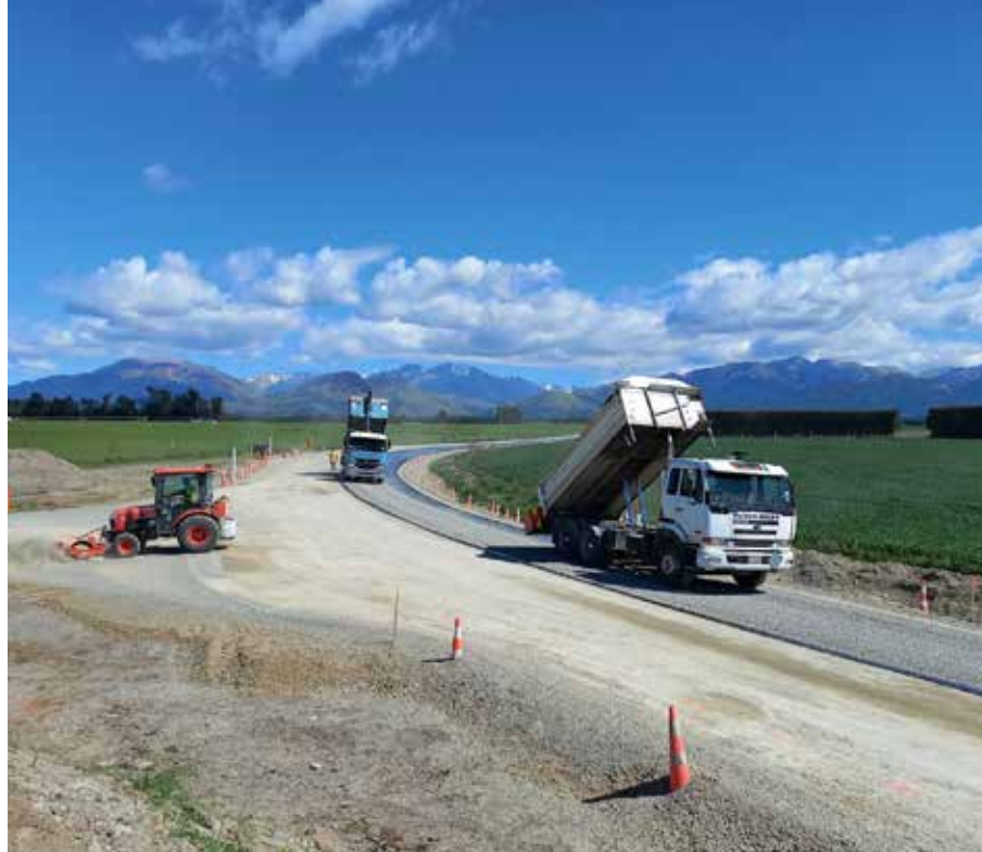
Rehabilitation work at Pudding Hill Road, Methven, has almost been completed.
