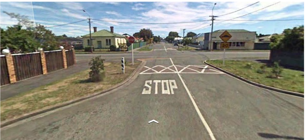
Figure 5 - Example of Intersection Throat Treatment.
