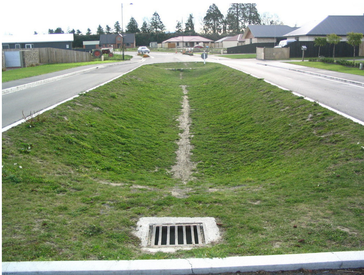
Figure 5-3 – An example of an infiltration basin / swale located within a central median
