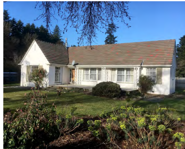
EXISTING CURATOR'S HOUSE
