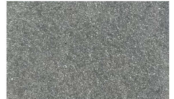
ACID ETCHED CONCRETE
