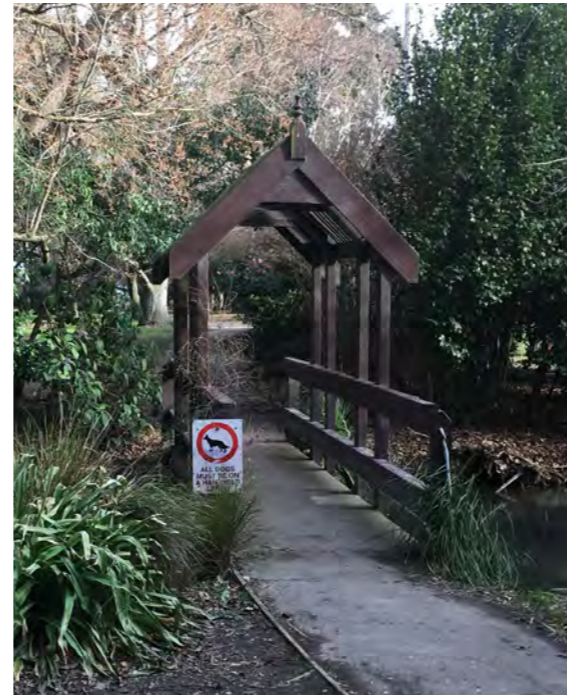
FOOTBRIDGE AT SPORTSFIELD END OF WATERWAY
